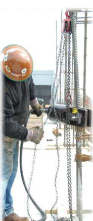
BarGrip XL cold—swaged coupling sleeves consist of seamless steel sleeves that slip over the ends of reinforcing bars. They are deformed onto the reinforcing bar profile to produce mechanical interlock.
